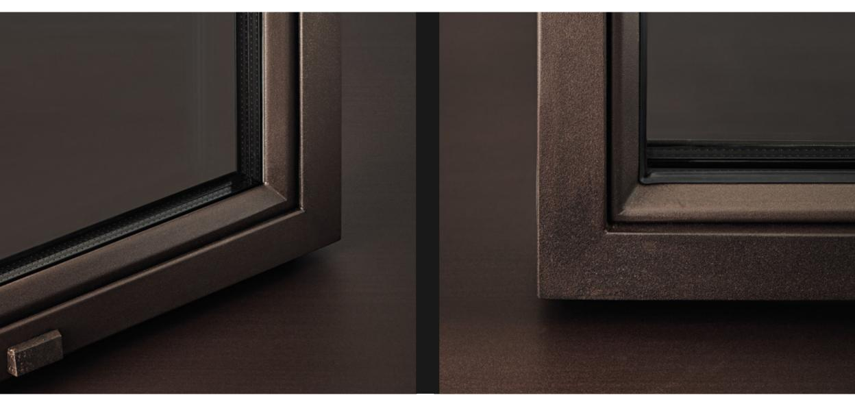
window corner in corten steel - external view window corner in corten steel with BV glazing bead - internal view
